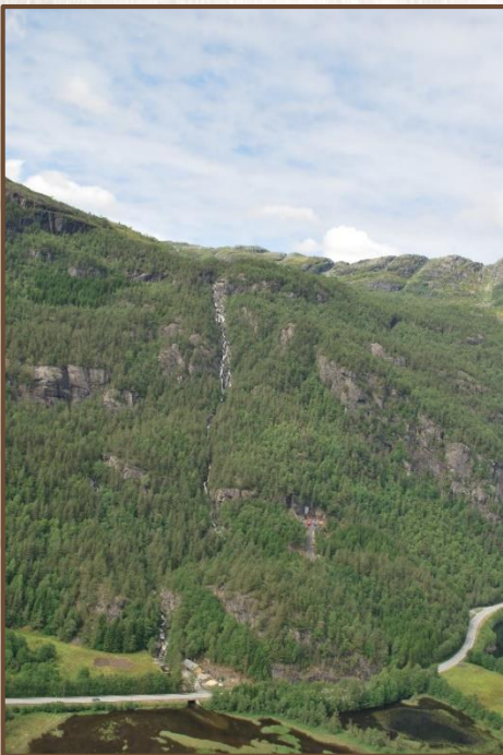
Archive photo of the completed Vågååna powerstation.
